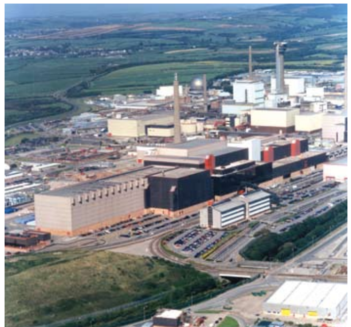
Thorp reprocessing plant © Sellafield Ltd
