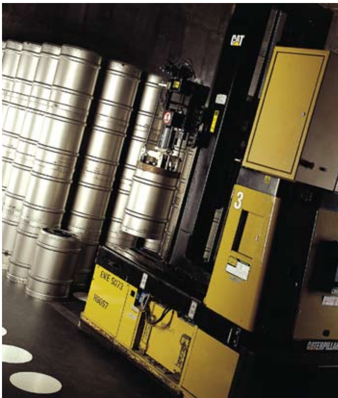
Uranium Oxide Storage Facility in Thorp © Sellafield Ltd
